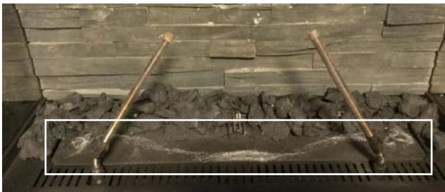
The "angel's hair" must be disentangled in length and deposit along the length of the burner according to the picture above.
